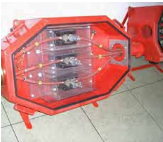
Special sealing end termination for Gothe-connection box
